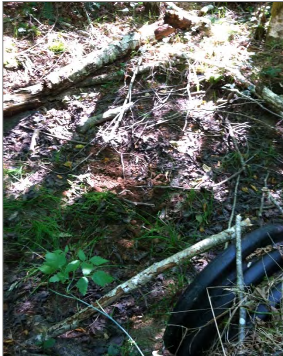
Photograph 4 Culvert outlet from Wetland J. Culvert is located under a gravel access road.
